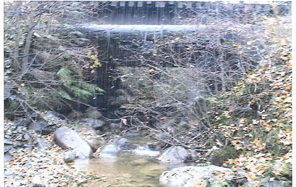
CK2308 From Downstream
