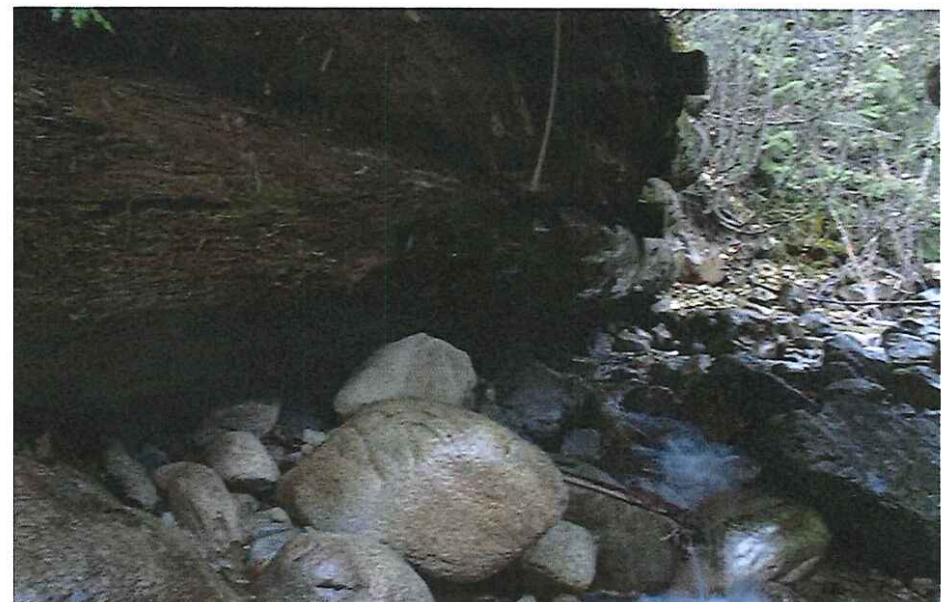
CK2308 Right Abutment Crib
