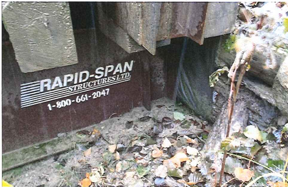
CK2308 Left Abutment Bearing
