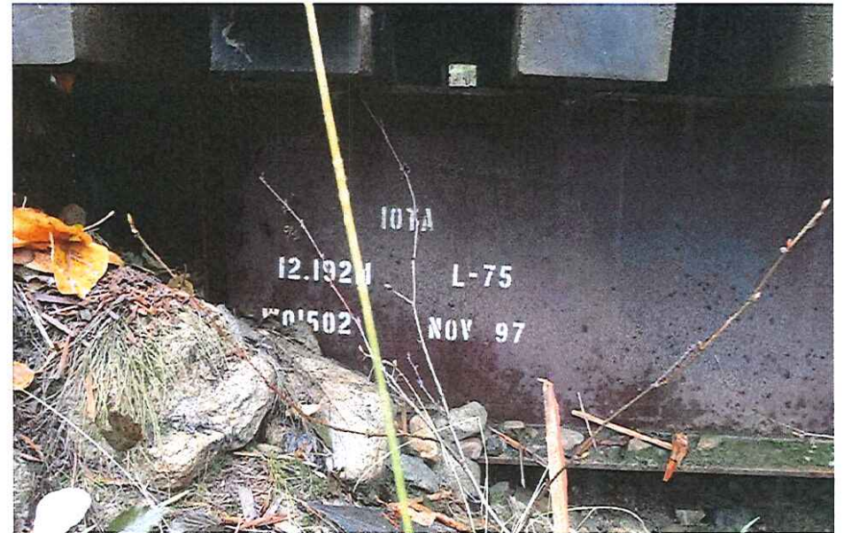
CK2308 Bridge ID
